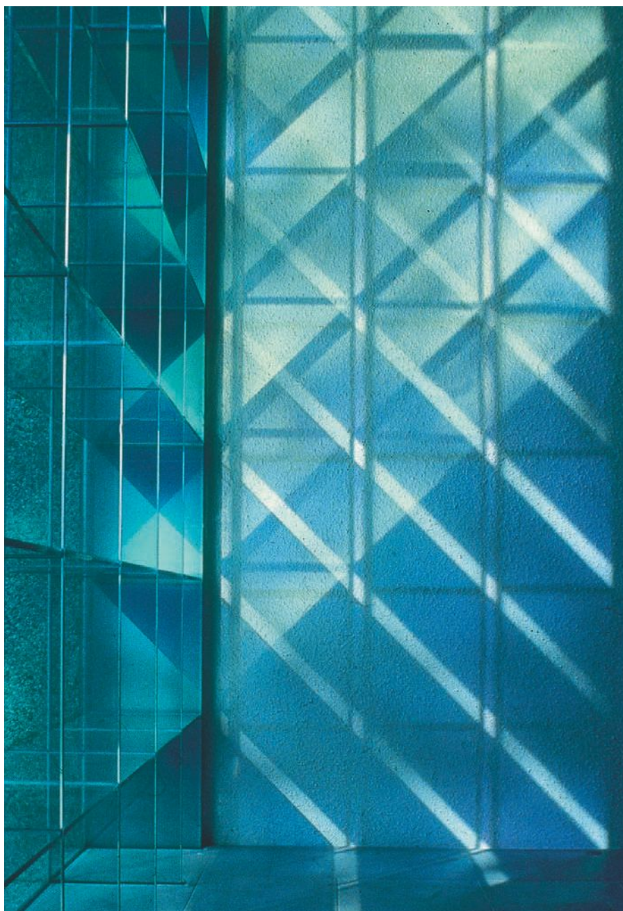
15 Flat glass and the diverse appearance forms of light: Church windows with a dichroic coating, Sweeny Chapel Indianapolis, 1987, Arch.: JCDA Inc.
