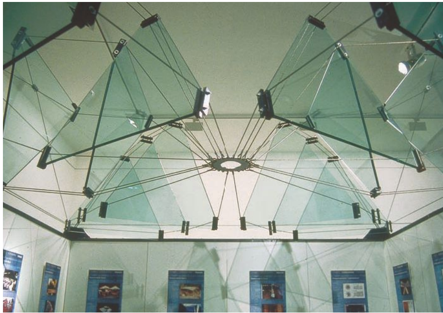
88, 89 Central tension ring composed of 3 mm stainless steel discs with a diameter of 210 mm
