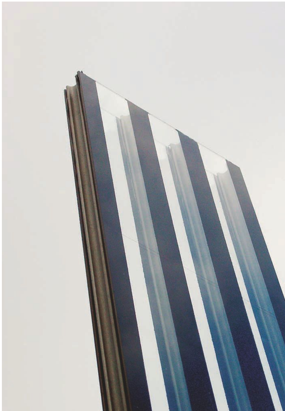
64 Insulating glass composite unit with integrated sun protection louvres, prototype with 3 m span
