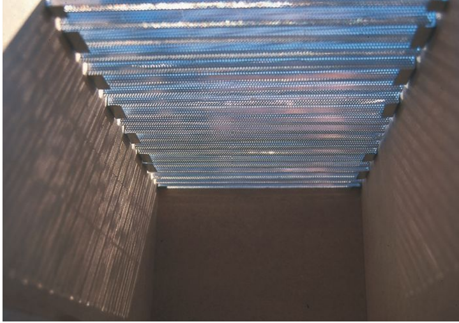
47 Bottom view of a roof structure with the steel-glass composite system across 15 m span; model project study "New Roofing for St. Pius X"
